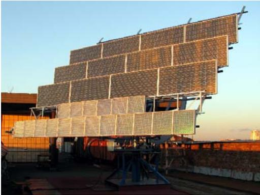
**Figure 14:** PV installation, which ensure appr. 5 kWp of output power (two lower rows – the concentrator modules; three upper rows – commercially available Si-based flat-plate modules).
