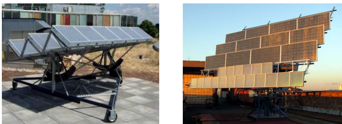
Fig. 4. On the left: PV installation with “carrousel”-type tracker and concentrator modules for 1 kWp of output power. On the right: PV installation with “tower”-type tracker, which will ensure appr. 5 kWp of output power (two lower rows – the concentrator modules; three upper rows – commercially available Si-based flat-plate modules).
